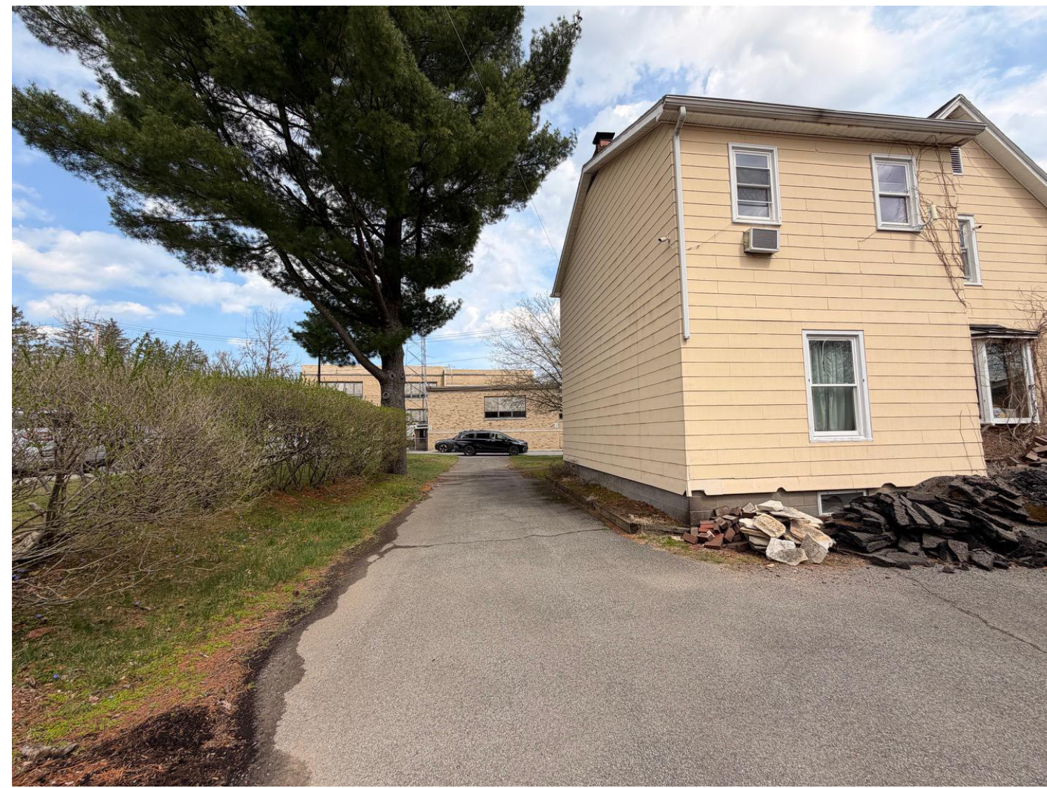
EXISTING ASPHALT DRIVEWAY
