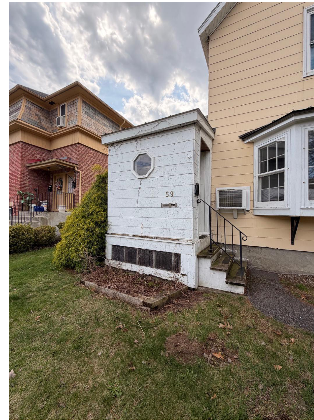
EXISTING ENTRY STAIR AND ENTRANCE
